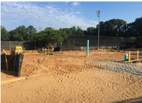
CSK- Sewer and Stormwater Cleanouts
