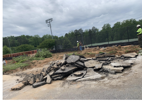
CSK- Pavement Demolition
